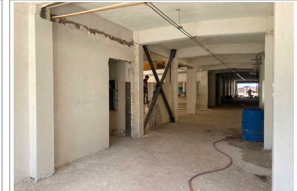
F5: Pasillo interior
